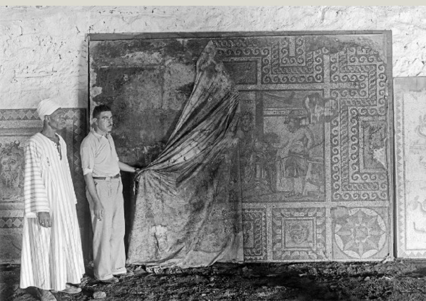
Barbari Mahmud Isa and William Gad Gabriel—foreman and supervisor, respectively, of the Antioch mosaic excavation crew—peel away muslin facing cloth from the Opora, Agros, and Oinos mosaic after removal from the House of the Boat of Psyche on August 24, 1934. Courtesy of Antioch Expedition Archives, Visual Resources Collection, Department of Art and Archaeology, Princeton University
